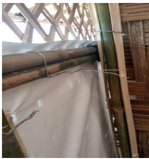
Do not cut off excess GI ware
