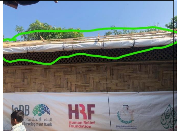
Right roof tarpaulin set with Mua
