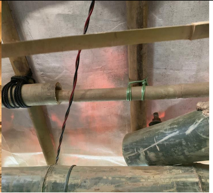
Comparatively thin and insect biting muli used.
