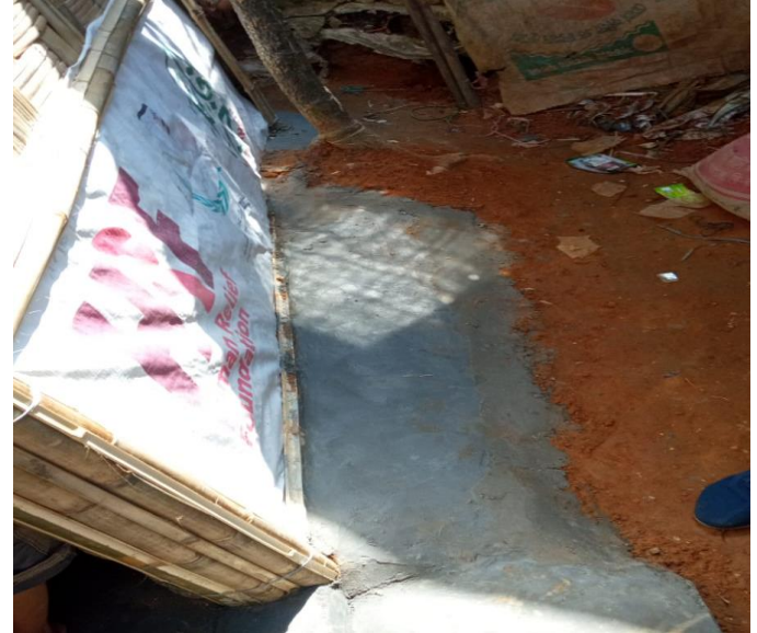
GEO bag not found in the outside plinth
