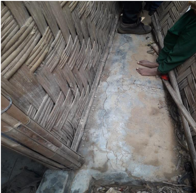
Cement plaster is not adjusted on GEO bags and GEO bags questionable setting around the plinth
