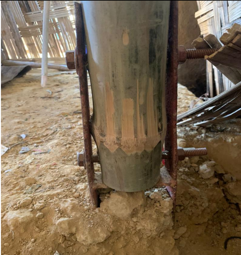
No gap between Boark and floor
