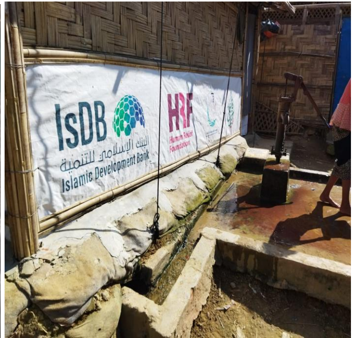
Cement plaster is not adjusted on GEO bags and GEO bags questionable setting around the plinth
