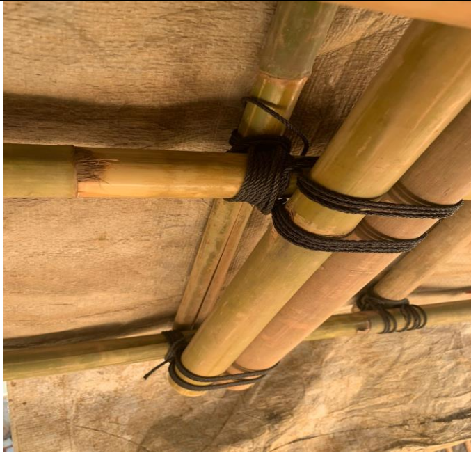
Immature muli bamboo used in the roof
