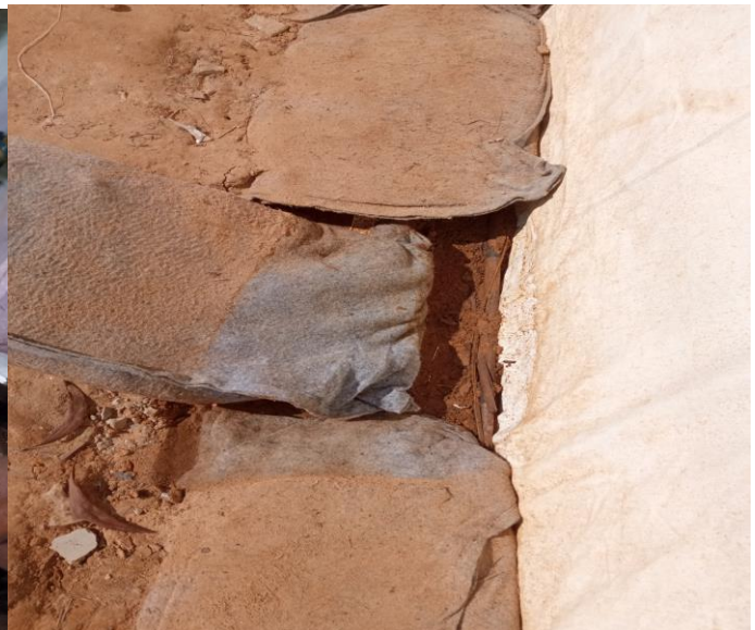
GEO bag set up in wrong methodologically
