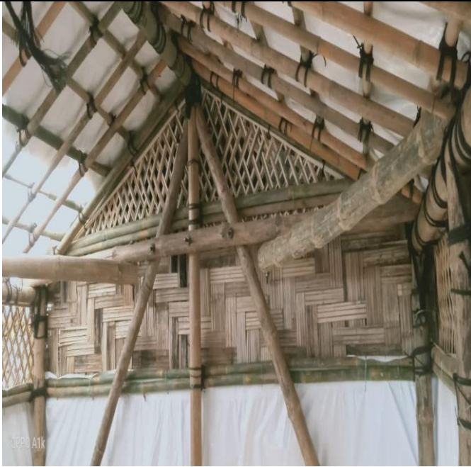
Less standard borak used in MTS construction
