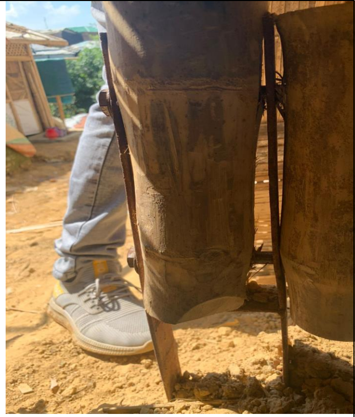
Wrong set of metal putting with Borak bamboo
