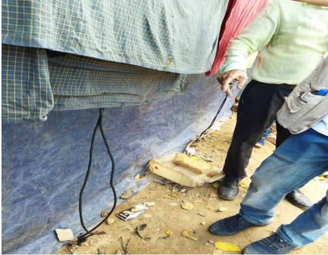
Loose tie down kit and not adjusted with MTS
